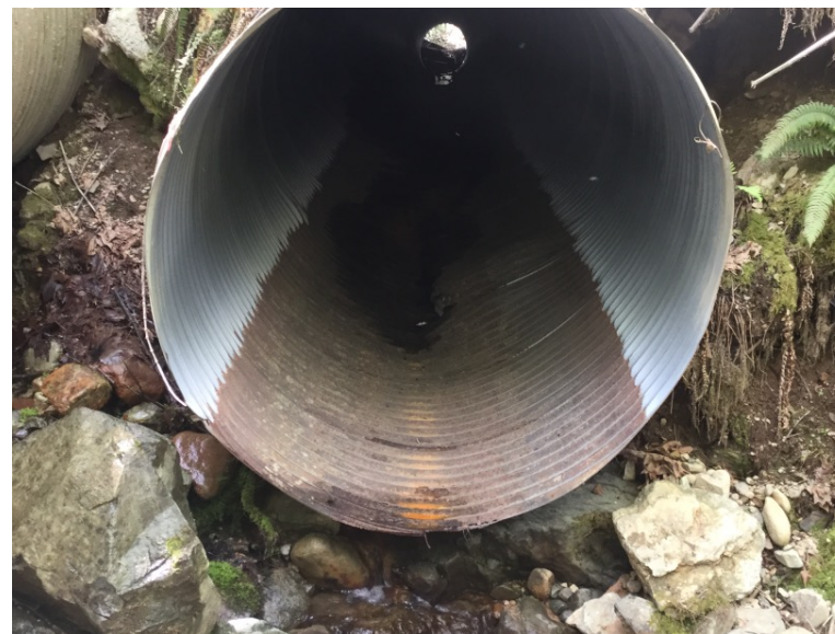
Outlet of upchain culvert
