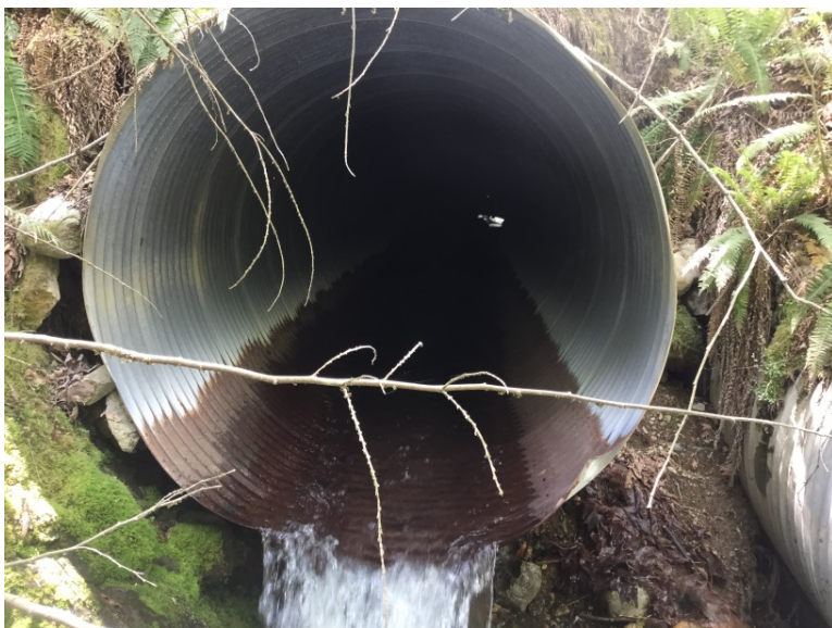
Looking through downchain culvert from outlet
