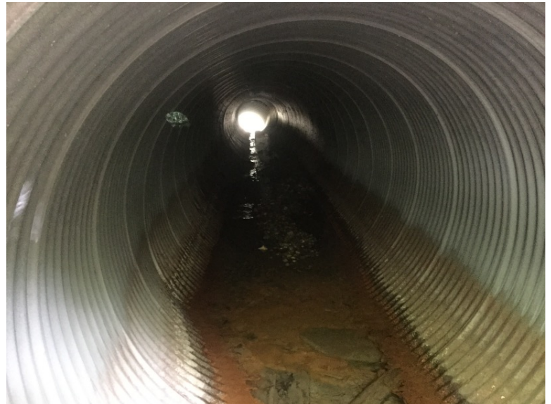
Looking through upchain culvert from inlet
